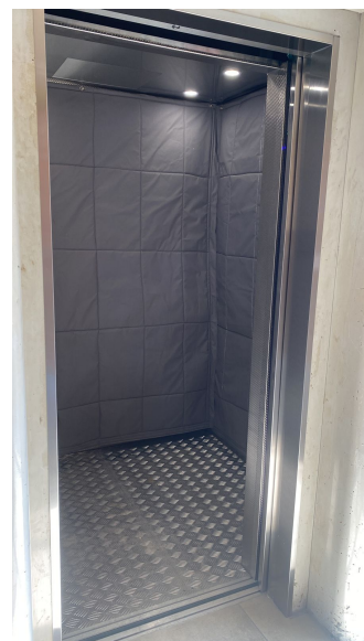
CBD RESIDENCY AJO BUILDING : NIDEC ELEVATORS
