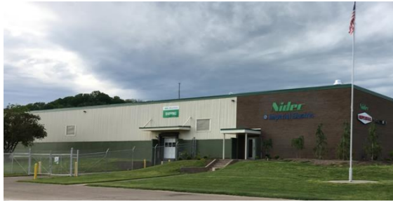
Nidec Imperial Electric, US, 1908 Elevator machine
