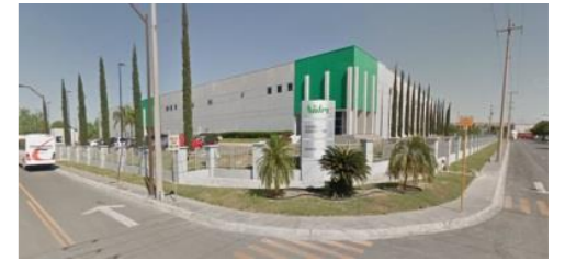
Nidec KDM, Mexico Elevator control system
